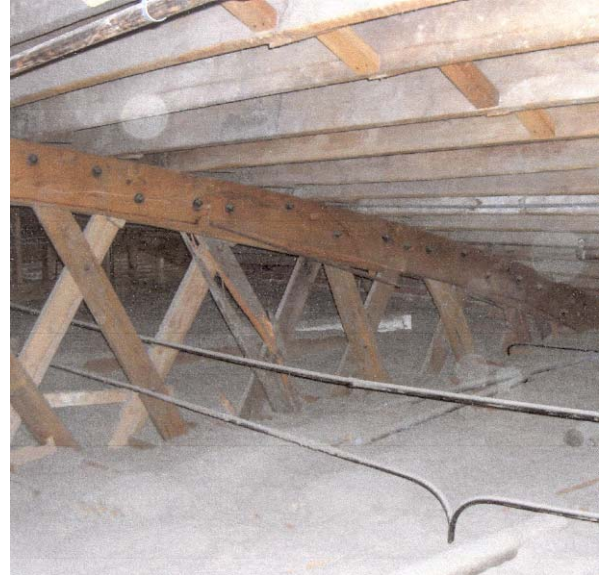
Grid G truss with visible broken structural members
