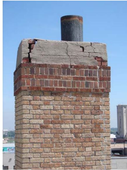
View of deteriorated cap
