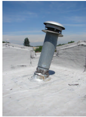
Mechanical flue penetration
