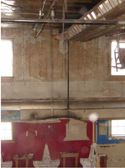
Grid line G sagging truss
