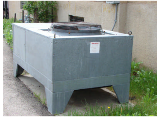
Condenser for Air Handler No.2
