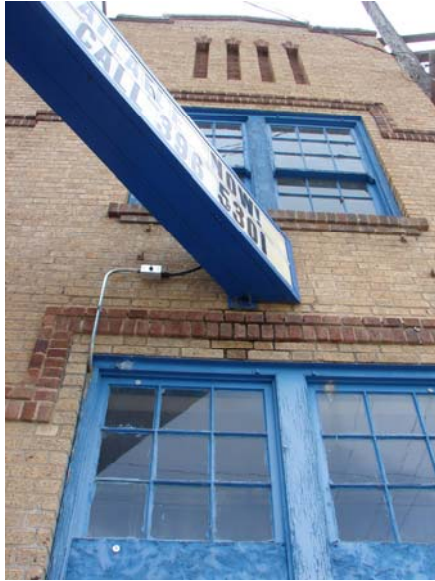
Sign connection at wall
