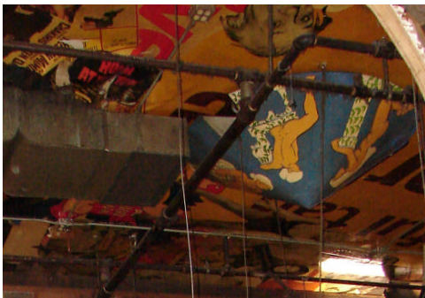
Typical suspended fire protection piping and heads
