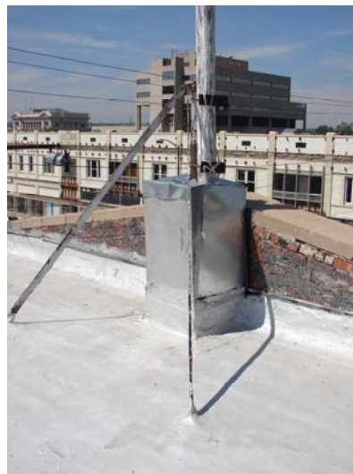
Flag pole roof top connection
