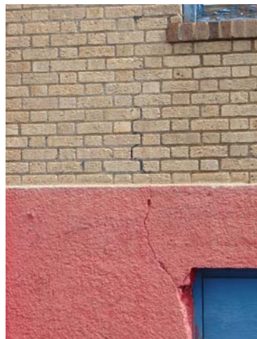
Exterior foundation wall crack at grid 1B (typical of 6 locations, all at window corners)
