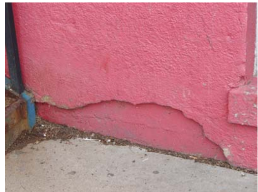
Exposed exterior foundation wall- grid 3A exhibiting some slight cosmetic cracking
