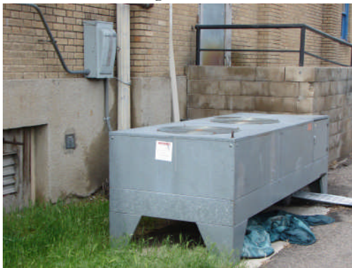
Condenser for Air Handler No.1
