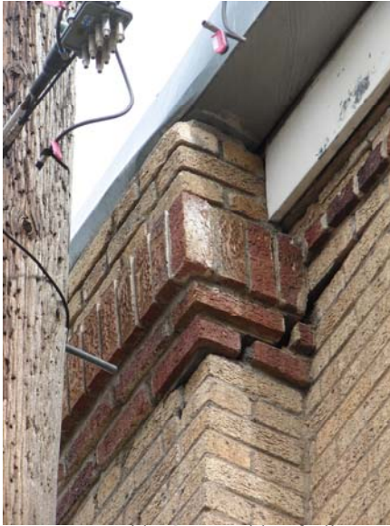
Damage at grid 1G-East side of pilaster
