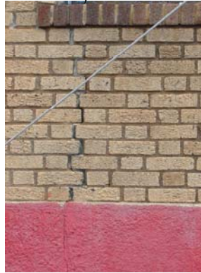
Cracks at window corners- typ. of 6 Grids E-H on both North and South Facades
