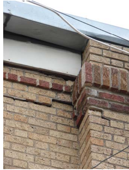
Damage at grid 1G- West side of pilaster
