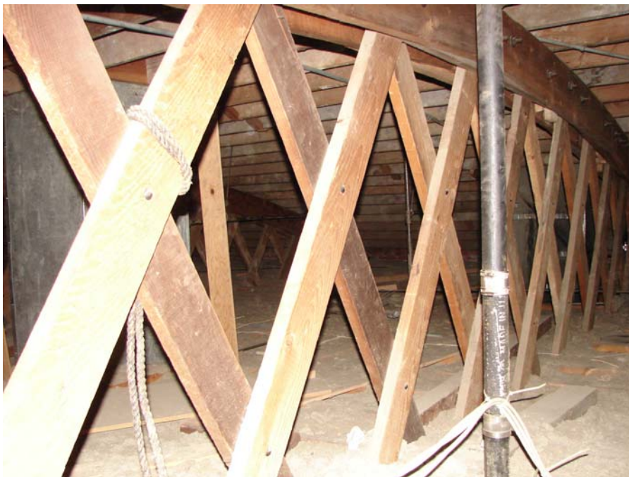
Typical truss configuration and web member layout
