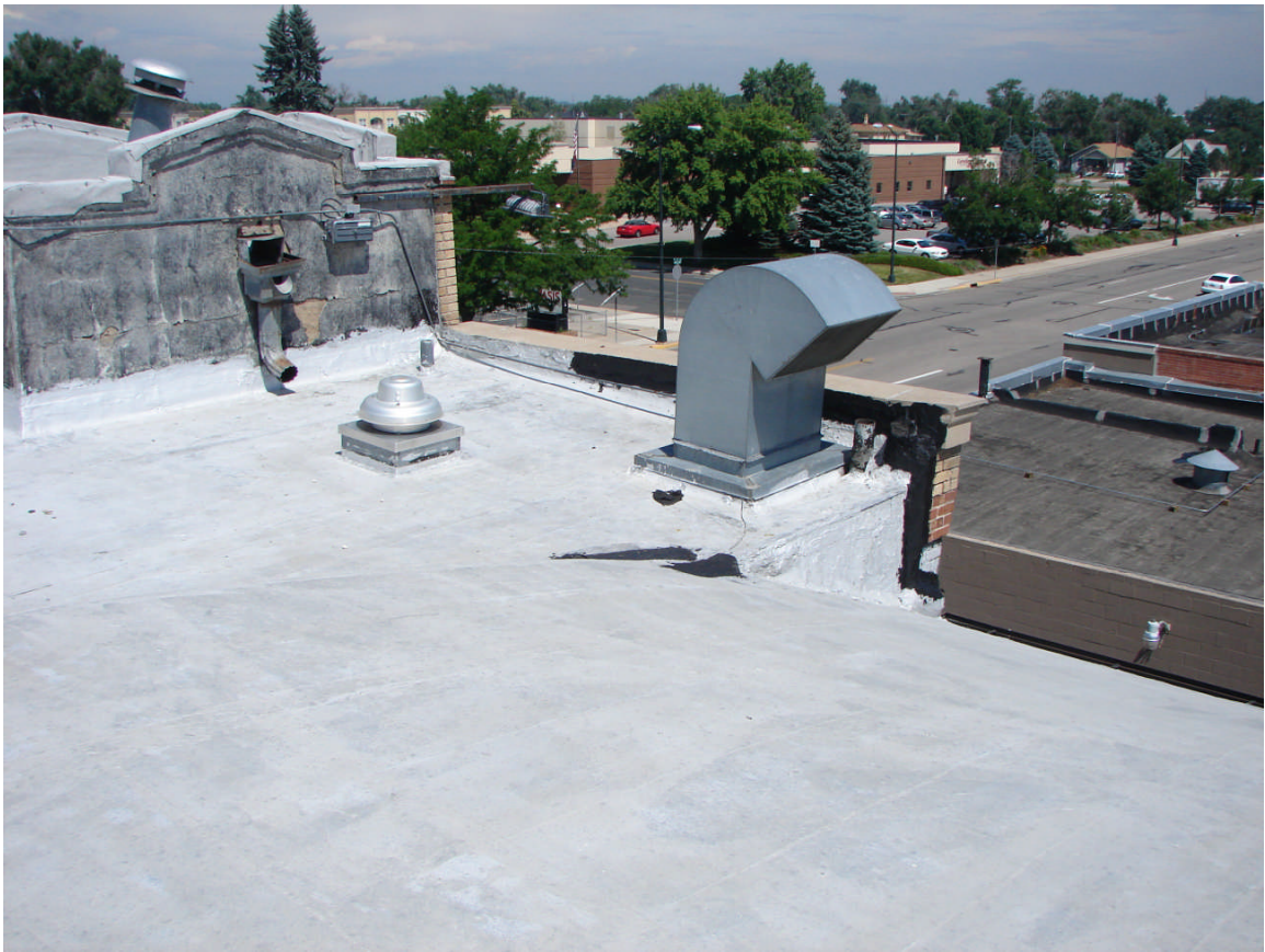
Location of leak where fresh tar has been applied at the vertical transition
