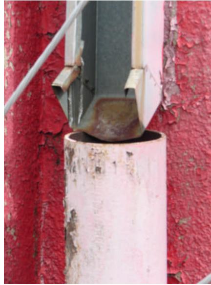
Downspout connection to storm~ grid 1H
