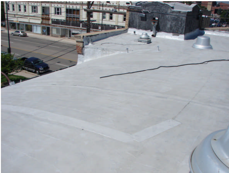
Patching and buckling of roofing felts
