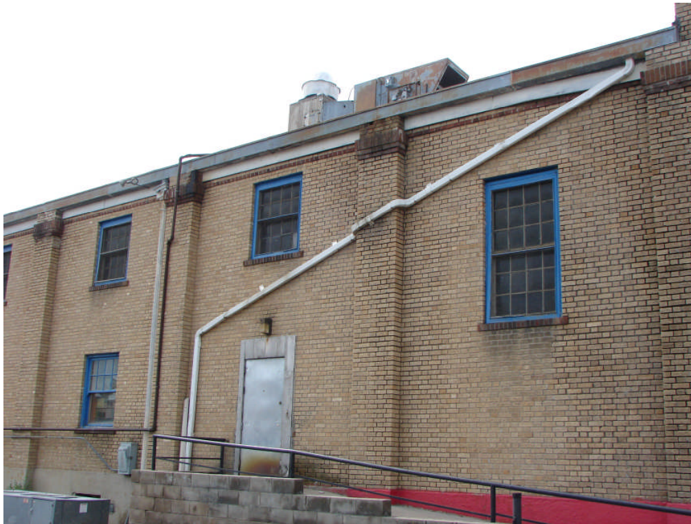
North façade downspouts and gutter system
