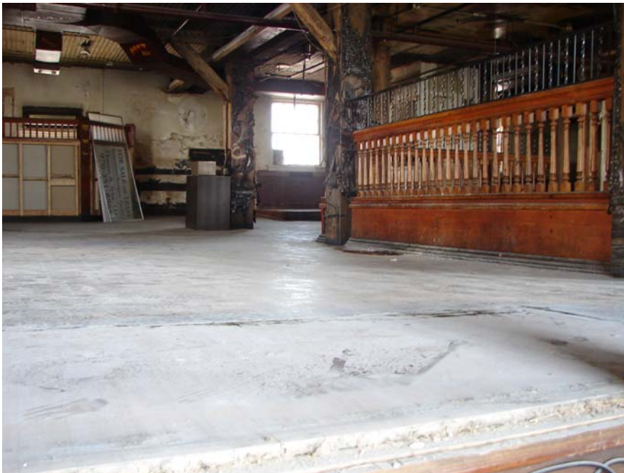
Sloping Mezzanine floor along grid D~ water in low spot visible
