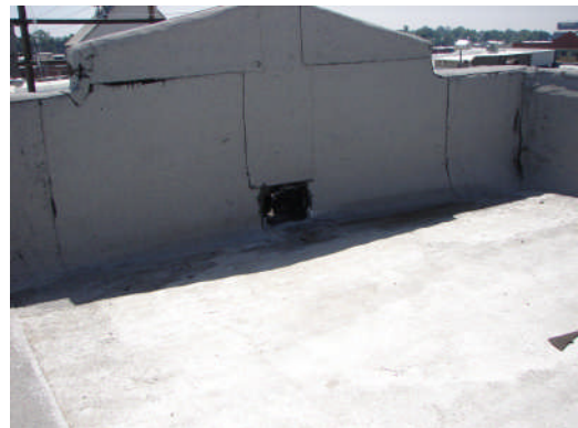
Typical Tower flat roof and scupper inlet
