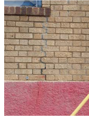
Cracks at window corners- typ. of 6 Grids E-H on both North and South Facades
